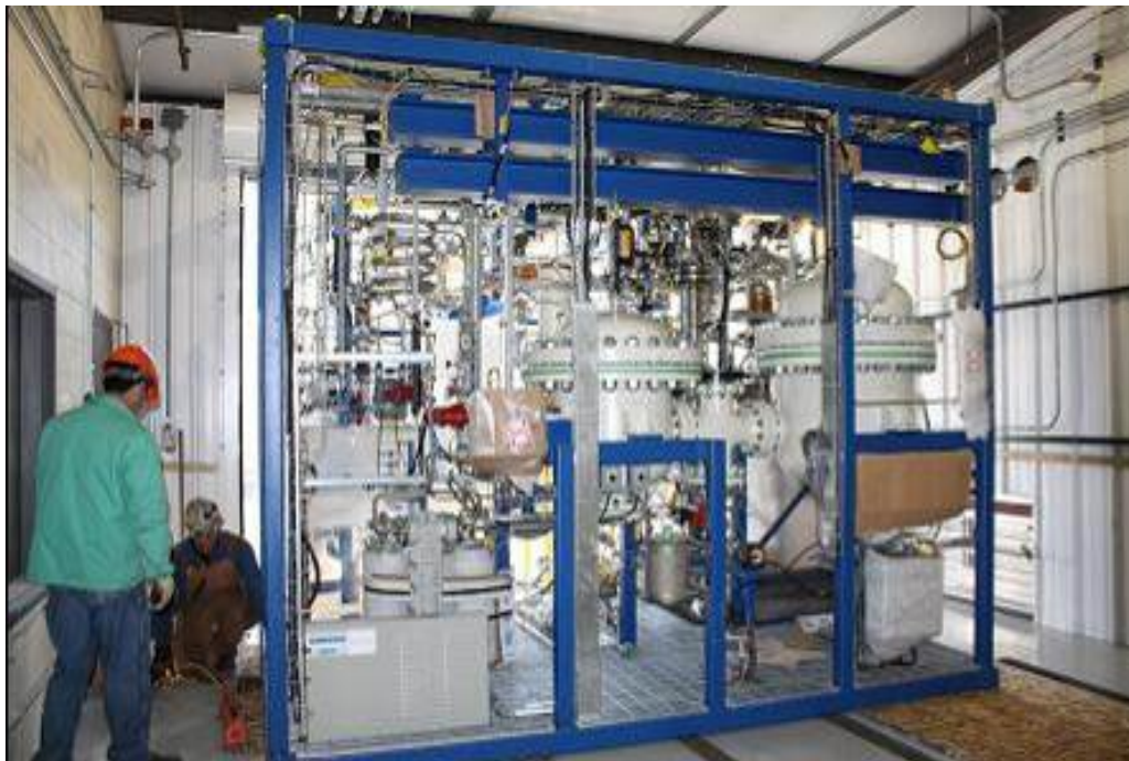
Figure 25—IH 2 Pilot Plant being slid into place
