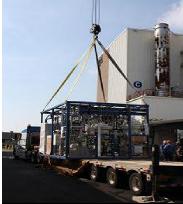
Figure 24—New 50 kg/d IH 2 Pilot Plant - lifted into place
