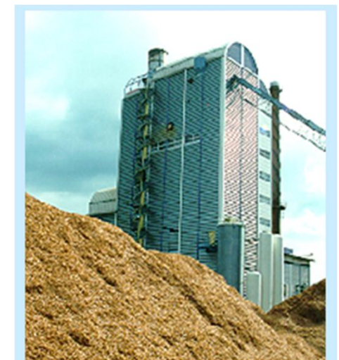
Biomass IGCC Demonstration Plant, Värnamo, Sweden
