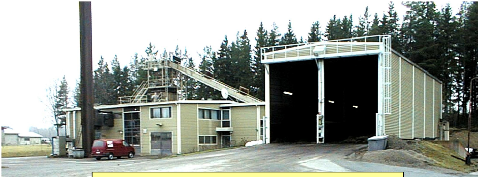
5 MW district heating plant, Jalasjärvi, Finland, in operation since 1987
